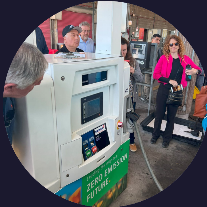
Hydrogen fueling pump
